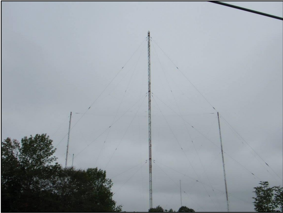
The three 550 foot towers that support the LF transmit antenna.
