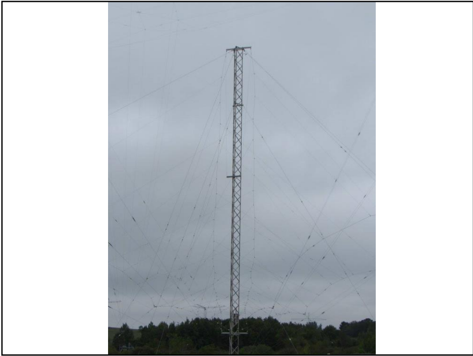
Omni-directional HF Log Periodic antenna.
